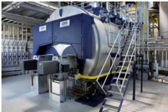
One UNIVERSAL ZFR double-flue boiler for saturated steam, steam output 30,000 kg/h, pressure 22 bar
