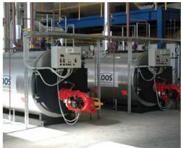
Two UNIVERSAL high-pressure steam boilers U-HD for saturated steam generation
