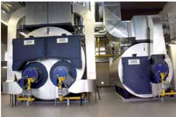
One UNIVERSAL ZFR double-flue boiler and one UNIVERSAL UL-S single-flue boilers for saturated steam, total system output 50,000 kg/h, pressure 16 bar
