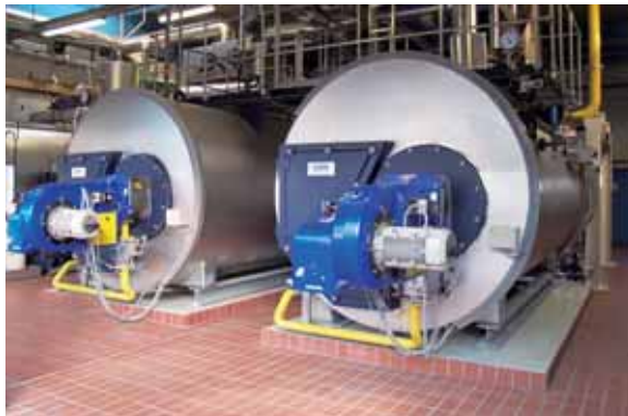
Two UNIVERSAL UL-S single-flue boilers for saturated steam, total system output 8,000 kg/h, pressure 13 bar
