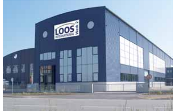
State-of-the-art manufacturing plant 2 in Gunzenhausen – production of shell steam boilers
